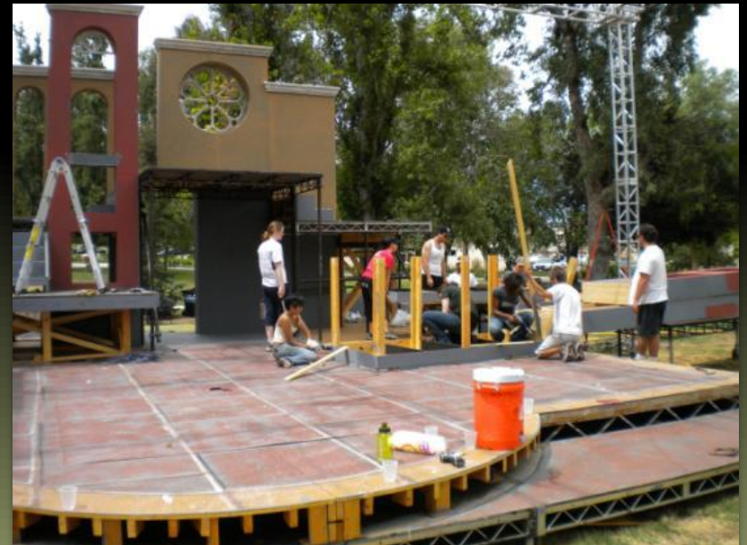
Stage with masonite deck and half-circle plug
