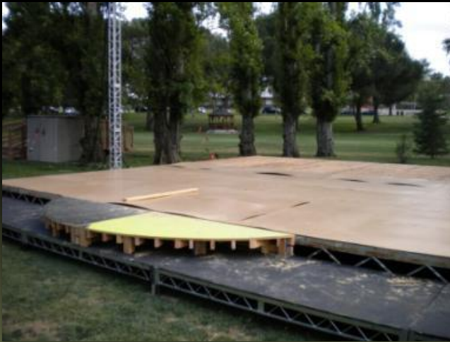
Stage with masonite deck and half-circle plug
